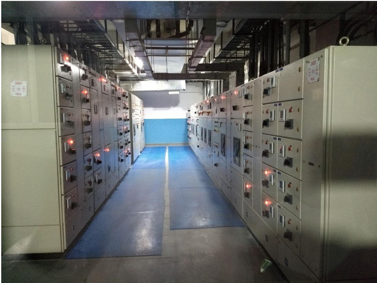
Main PCC Panel & Critical Load Panel
