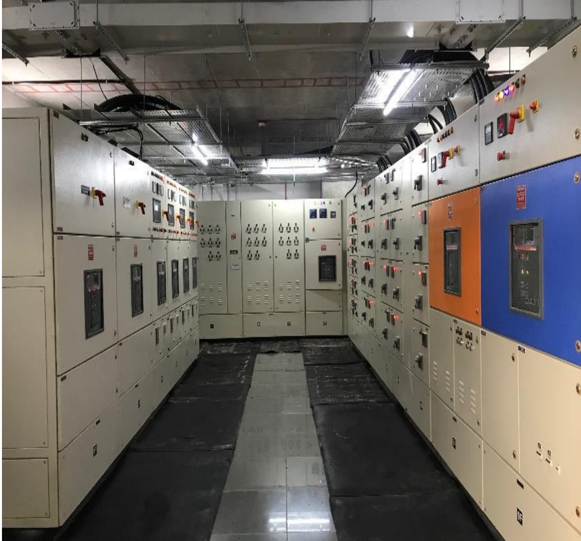
Main PCC Panel + APFC Panel & 4 x 500 KVA Gensets' Synchronizing Panel connected with BBT
